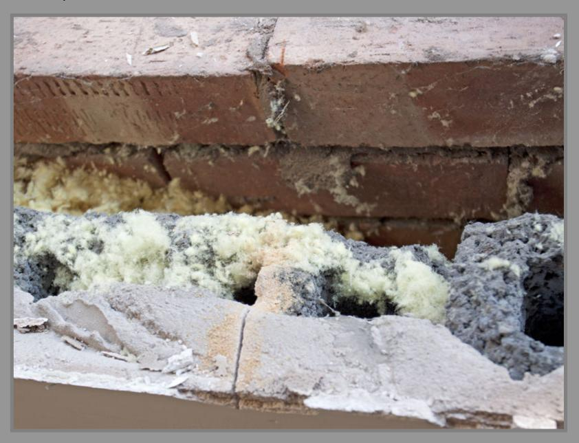
This second image is of the void viewed from inside the house and is therefore on the right of the window. The line of insulation falls away at a steep angle about 200mm from the end. The void is variable obviously but at the deepest point 640mm from the top edge of the brick. Image taken immediately the void was discovered. Not acceptable especially as I was at the time carefully fitting a new uPVC window with B rated frames and K glass (fully compliant).
